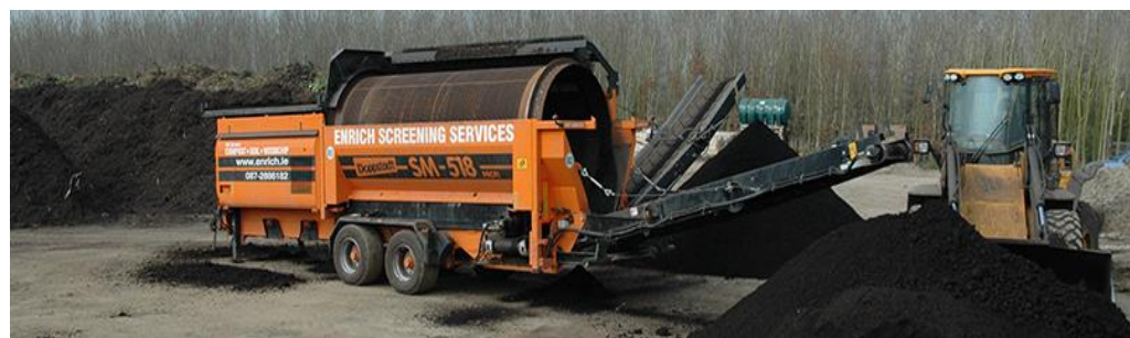
Figure 4: Fine screening compost on-site.
