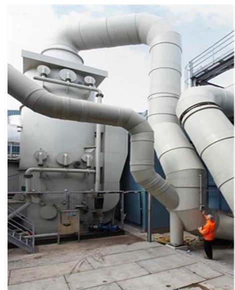
Figure 2: Acid air washer for Ammonium sulphate production.
