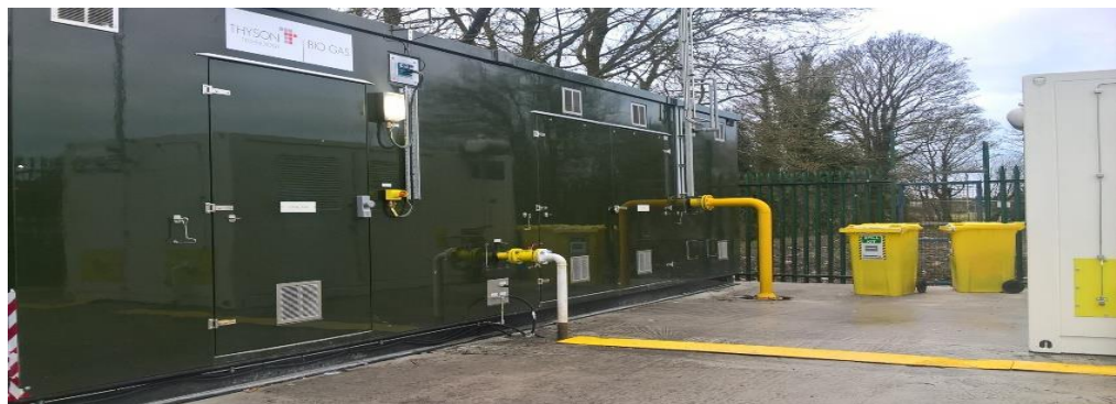
Figure 4: The modular grid entry unit and the gas quality monitoring and metering of biomethane unit at the Cush site.
