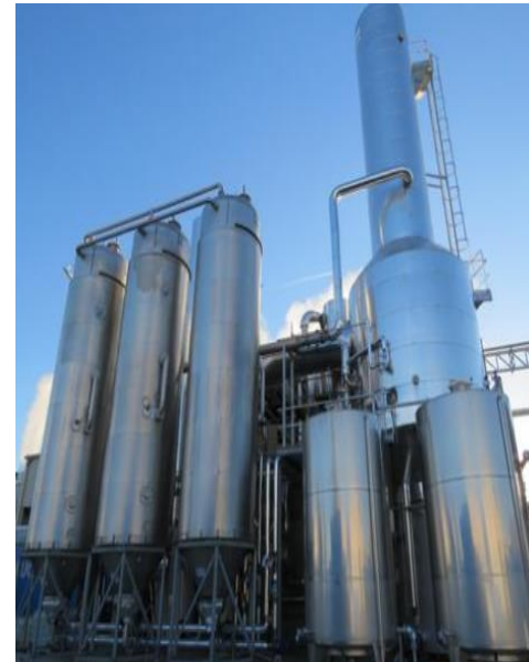
Figure 3: Evaporators at Kallo location of Group op de Beeck.
