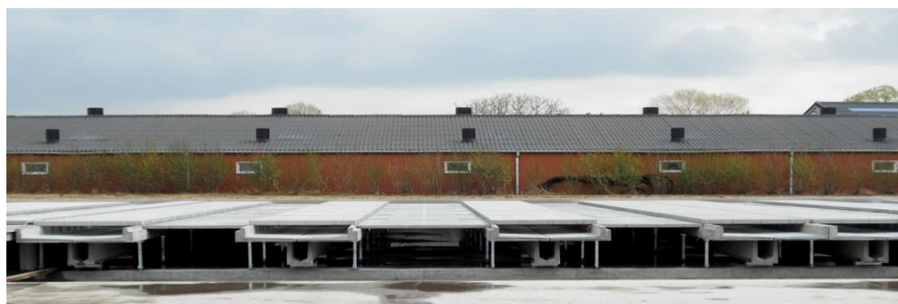
Figure 3: Installed VeDoWS system at an animal stable.
