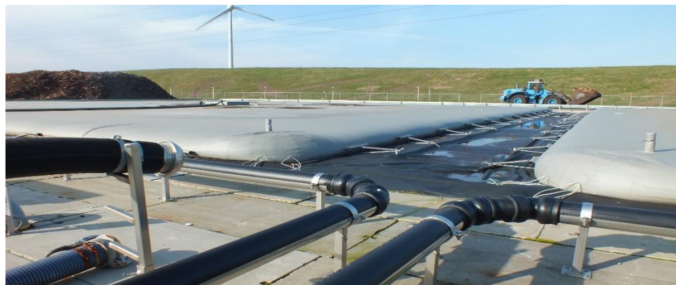
Figure 3: Storage bag tanks for Ammonium sulphate.
