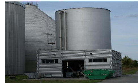
Figure 2: AirPrex® - plant in Berlin-Waßmannsdorf
