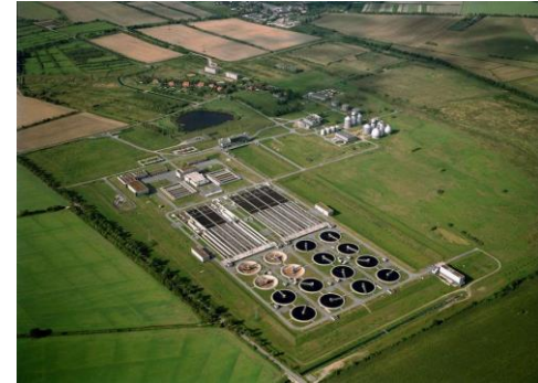
Figure 1: Waste water treatment plant in Berlin-Waßmannsdorf
